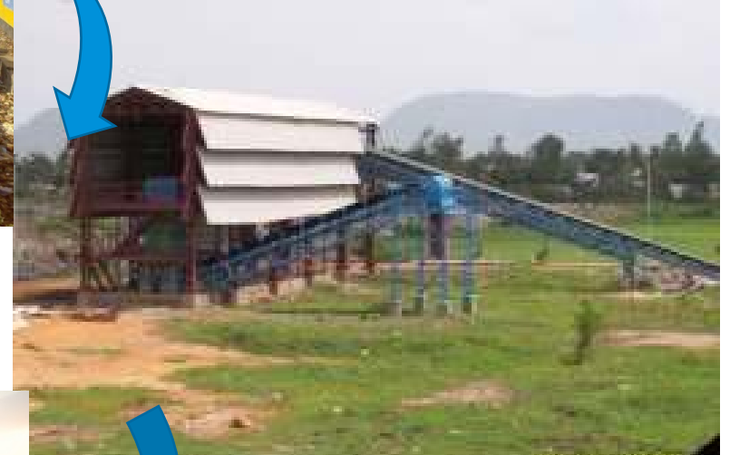
Segregation/Waste to Energy Processing Facility
